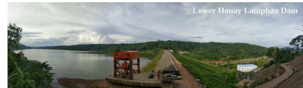
Lower Houay Lamphan Dam Grouting
